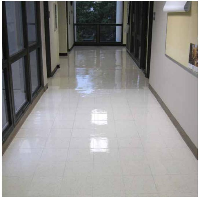
The final result of the case study can be seen above. The yellowed floor was stripped with Pry-Bar Floor Stripper, neutralized with Envision Neutral Floor Cleaner and coated with Tough As Nails Green Floor Coating. The differences are apparent. The result: Momar's "Green" floor care products produced a brilliant shine and gave the floor a glossy, "wet" look that will withstand gloss-killing dirt, grit, and sand.
